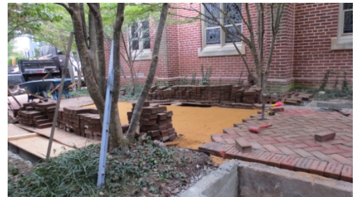
Re-laying the brick walk
